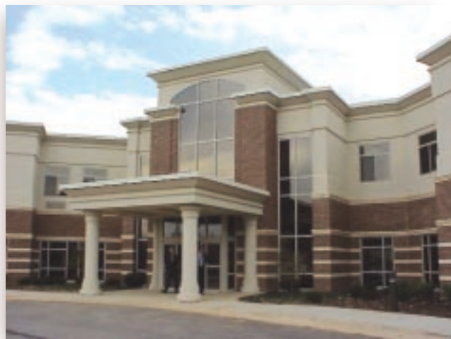
Kessler Adventist Rehabilitation Hospital, Rockville, Maryland
